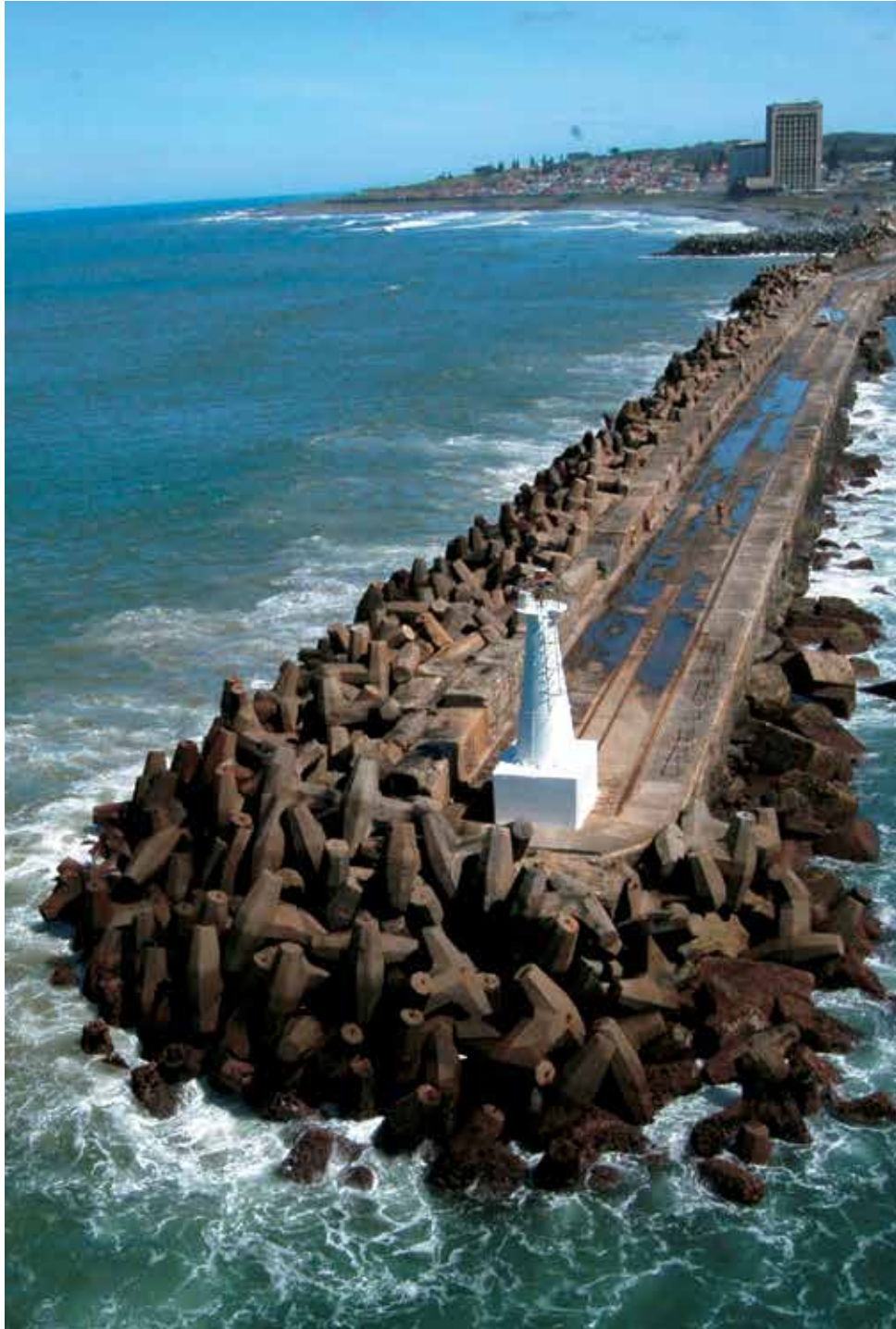
The East London main breakwater with dolos protection. The structure is approximately 600 metres in length from west to east at the mouth of the Buffalo River. Each dolos consists of 20 tons of concrete. The CSIR carries out annual monitoring surveys to assess the stability of the breakwater for Transnet.
