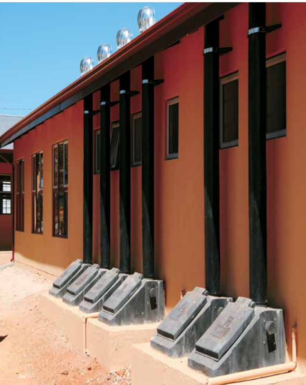
The Myra Primary School in Taung in North West was completed using innovative building technologies. The structures against this wall form part of an off-grid sanitation system.
