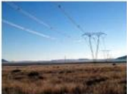
765kV Transmission Pylon @ 1000m
