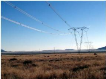
765kV Transmission Pylon @ 500m
