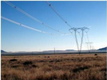
765kV Transmission Pylon @ 500m
