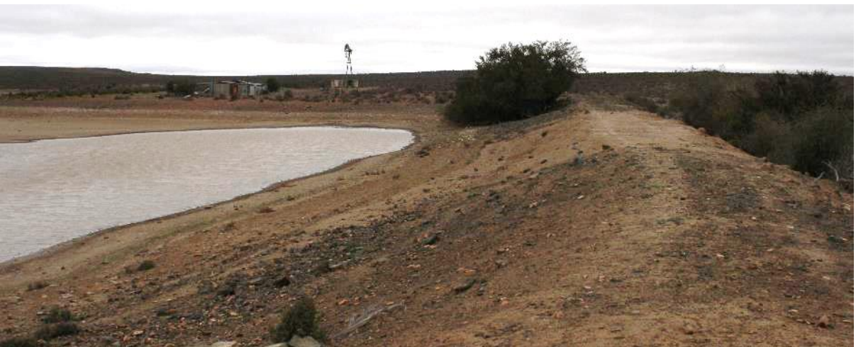
Figure 3: A ground dam
