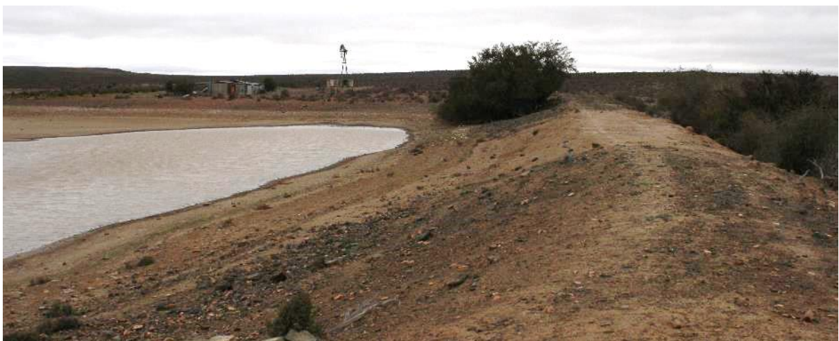
Figure 3: A ground dam
