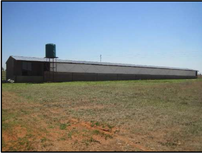
Figure 6. General Site conditions – existing chicken house.
