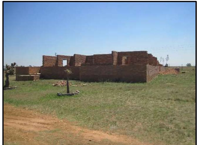
Figure 9. General site conditions – existing structures.
