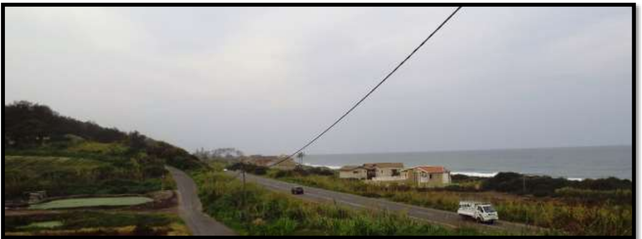
PROPOSED PIPELINE TUNNELS BELOW M4 MOTORWAY AND UNDER TERTIARY DUNE CORDON TO BEYOND SURF ZONE (1)
