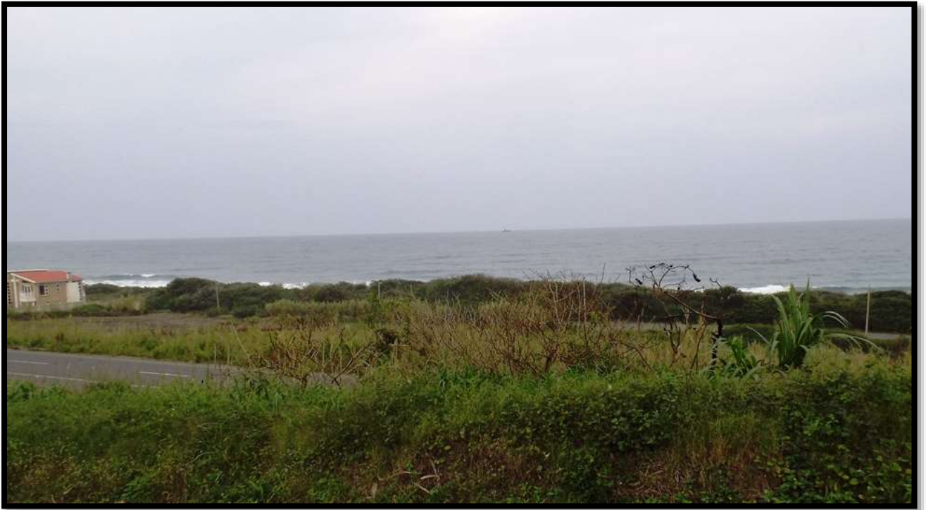
PROPOSED PIPELINE TUNNELS BELOW M4 MOTORWAY AND UNDER TERTIARY DUNE CORDON TO BEYOND SURF ZONE (2)
