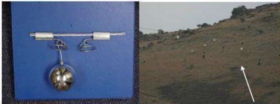
Figure 5: A Reflective Bird Diverter (left) installed on a line with conventional bird flappers (right).
