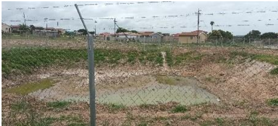
Figure 2: Stormwater (Detention Pond)
